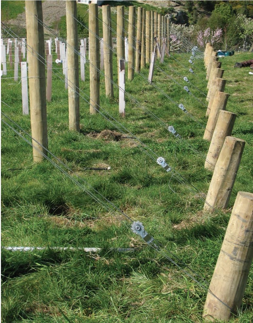
Fig. 6.26. Tieback end assemblies. Two loops of wire are used to link the strainer to the end post and each has a wire tensioner to adjust the strain on the posts.
