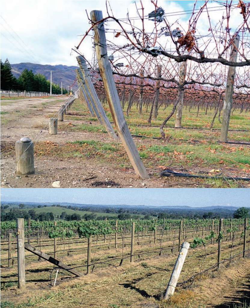
Fig. 6.29. Top: an end post that is not strong enough to withstand the tension of the wires ties to it. Bottom: a free-standing end post that has failed due to inadequate strength. The adjacent row has already been retrofitted with a diagonal stay assembly in recognition of the original oversight.
