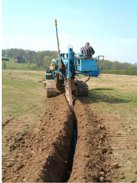
Drainage machine laying drains before planting
