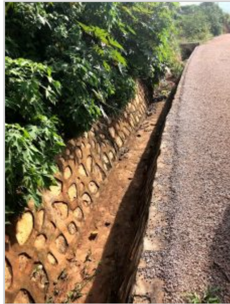
This road ditch in Uganda has completely covered the area water would run with cement and rocks so it cannot erode and undermine the road. Photo Credit: Amber Anderson.
