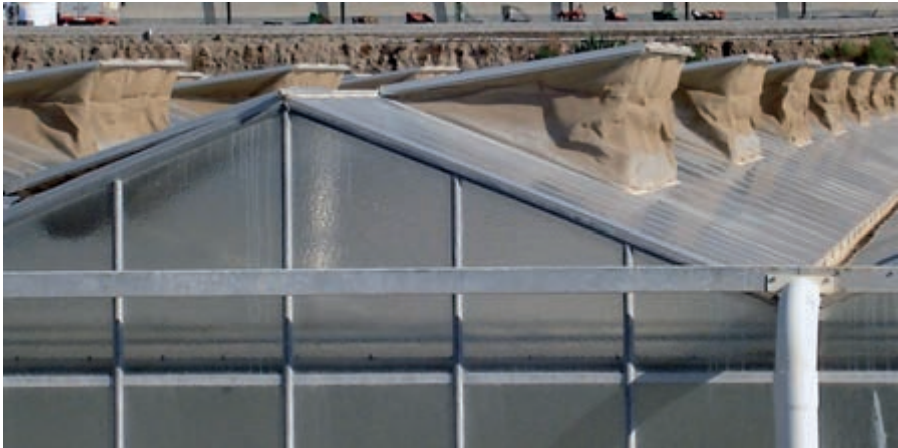
Figure 55. Alternate windows in a Venlo greenhouse constructed in Almería
