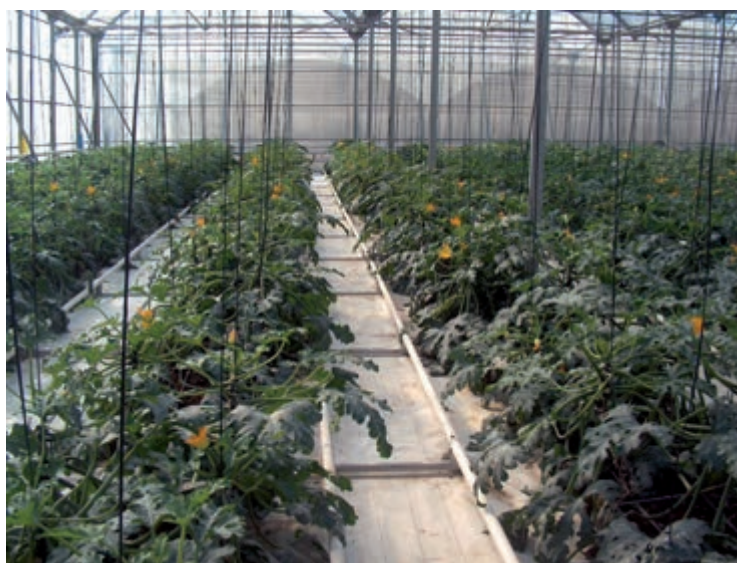
Figure 90. Heating system using metal pipes of hot water
