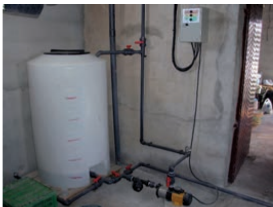
Figure 118. Fertigation system using a direct aspiration pump tan
