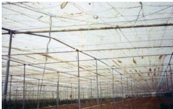
Figure 24. Inside of an older-type of flat-top greenhouse with a metal structure
