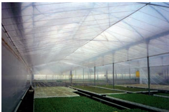
Figure 105. Installation of a double roof in a nursery
