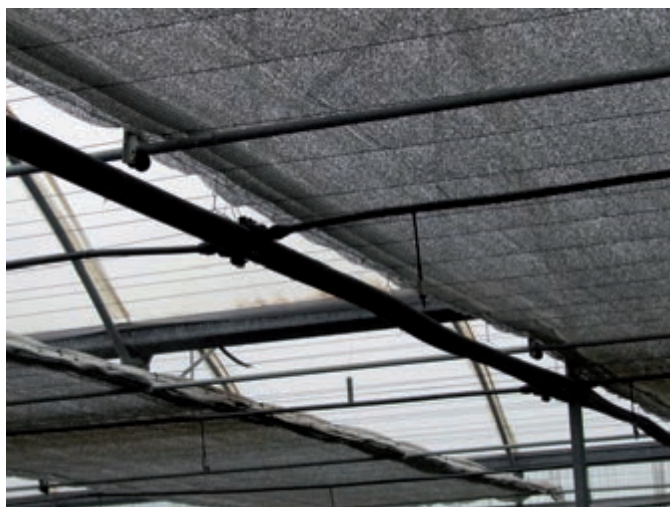
Figure 102. Double-sided aluminised thermal screen
