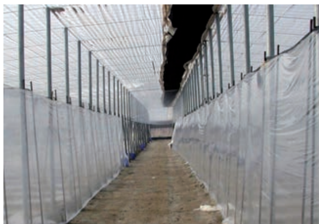
Figure 108. Interior partitions with polyethylene sheets inside a greenhouse
