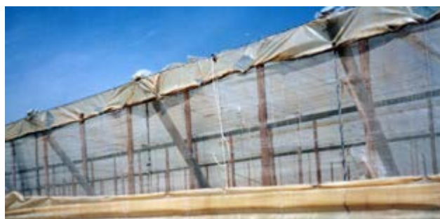
Figura 45. Sliding sidewalls with rope and pulley system
