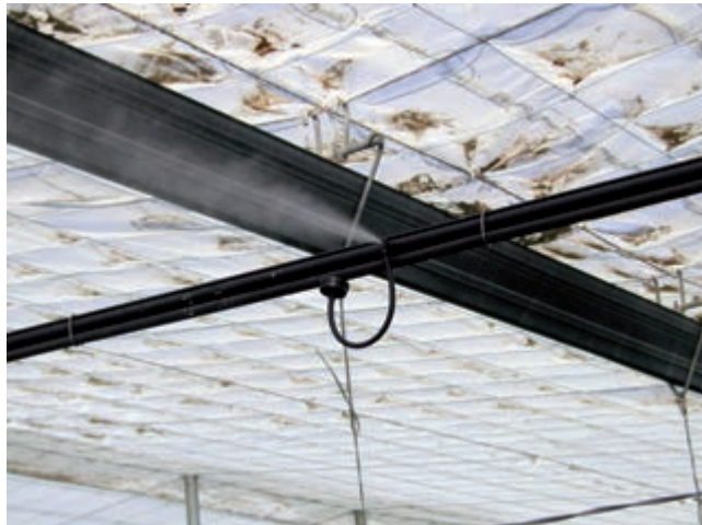
Figure 74. Detail of a fogging nozzle using compressed air in an Almería-type greenhouse
