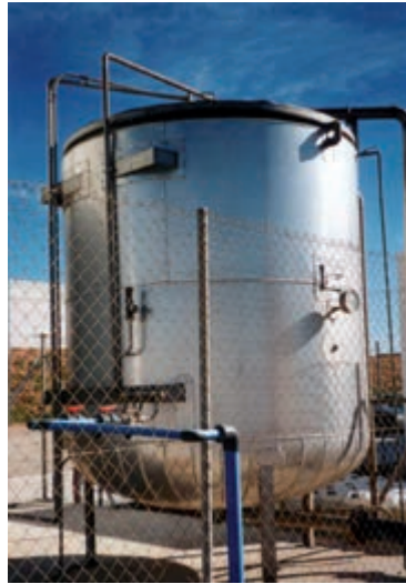
Figure 111. CO 2 evaporator with an auxiliary heating system
