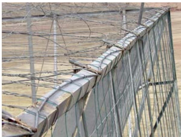
Figure 27. ‘Raspa y amagado’ greenhouse under construction
