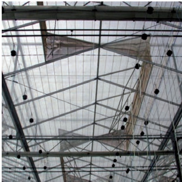
Figure 56. Interior view of discontinuous windows in a Venlo greenhouse
