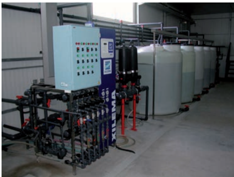
Figure 121. Automated fertigation system with Venturi injectors
