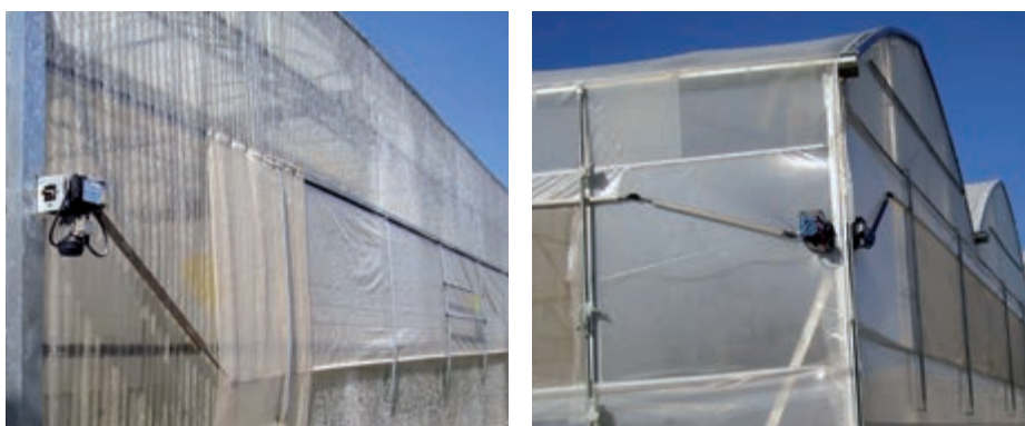
Figure 48. Roll-up side windows in multi-span greenhouses
