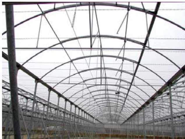
Figure 32. Structure of a cylindrical covered multi-span greenhouse
