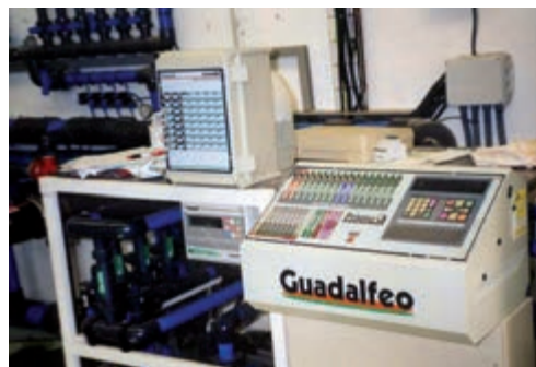
Figure 123. Electronic equipment of an automatic fertigation controller and a control panel with lights for the indication of operating systems
