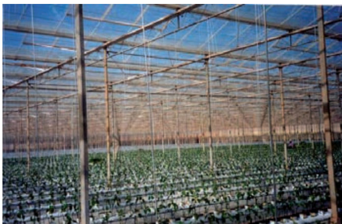
Figure 44. Venlo-type greenhouse in Almería
