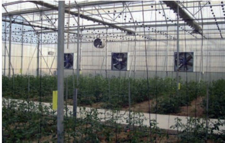
Figure 68. View of the fans located on the opposite band of the evaporator pads
