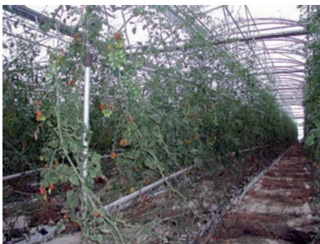
Figure 94. Heating system using hot water pipes of aluminium located at the height of the crop
