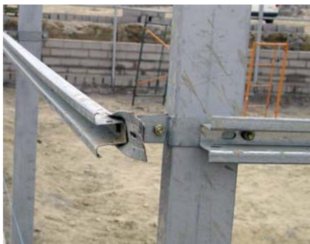
Figure 31. Omega profiles for the attachment of plastic in multi-span greenhouses
