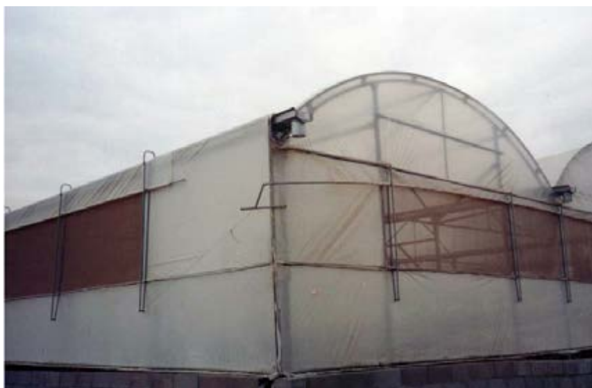
Figure 42. Multi-span greenhouse with polyethylene cover and sides
