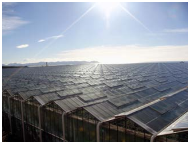
Figura 35. Venlo type greenhouse in Almería
