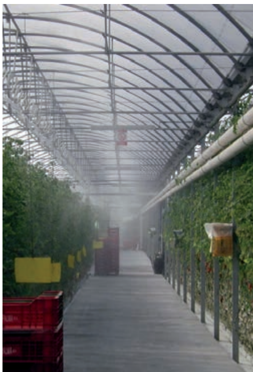
Figure 70. Mist created by a fog system
