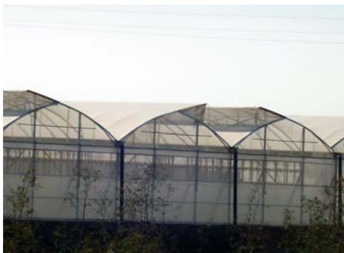
Figura 33. Gothic-type multi-span greenhouse with «superzenith» windows in the ridge
