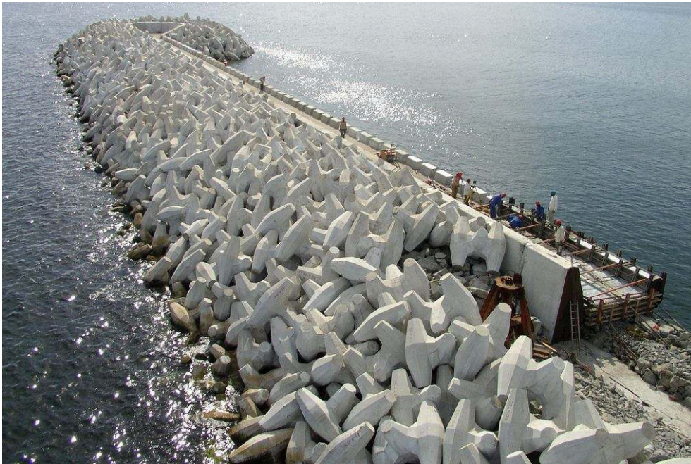
Fig. 33. Fujairah breakwater under construction (UAE)
