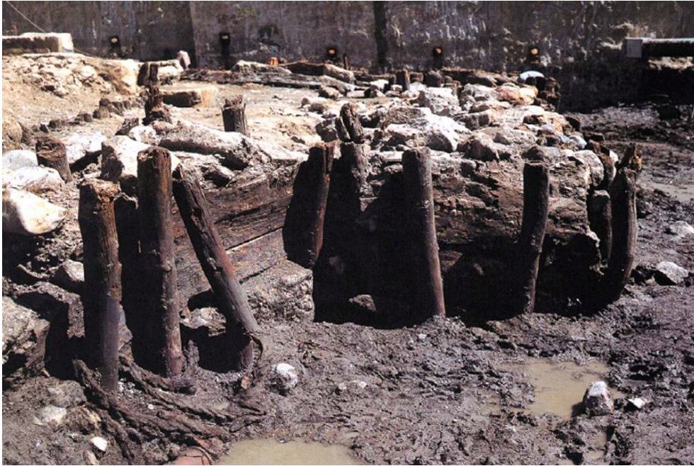
Fig. 22. Timber quay wall of place Jules Verne, Marseille
