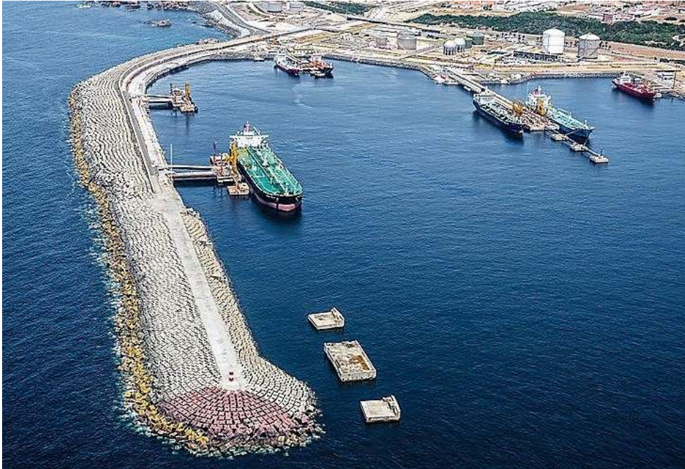
Fig. 34. Oil terminal on main breakwater at Sines (Portugal)
