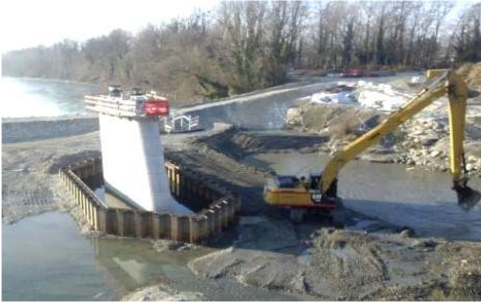
Fig. 29. Cofferdam for bridge pier in river Isère (France)
