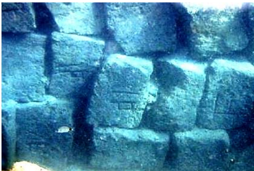
Built with ashlar headers (0.5x0.5x2 m) Noureddine, 2010
