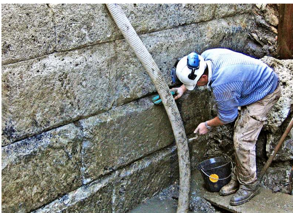
Built with ashlar stretchers Inrap, 2006
