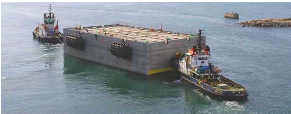
Fig. 12. 45 x 24 x 18 m caisson floated into position at Açú (Brazil)
