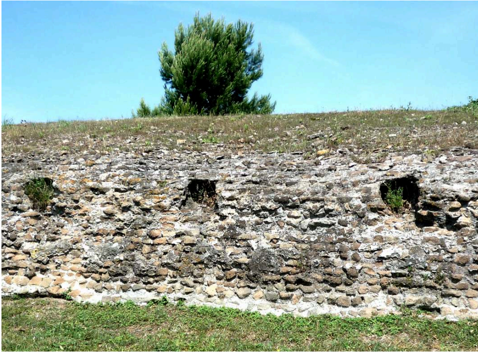
Fig. 5 - Portus' north breakwater
