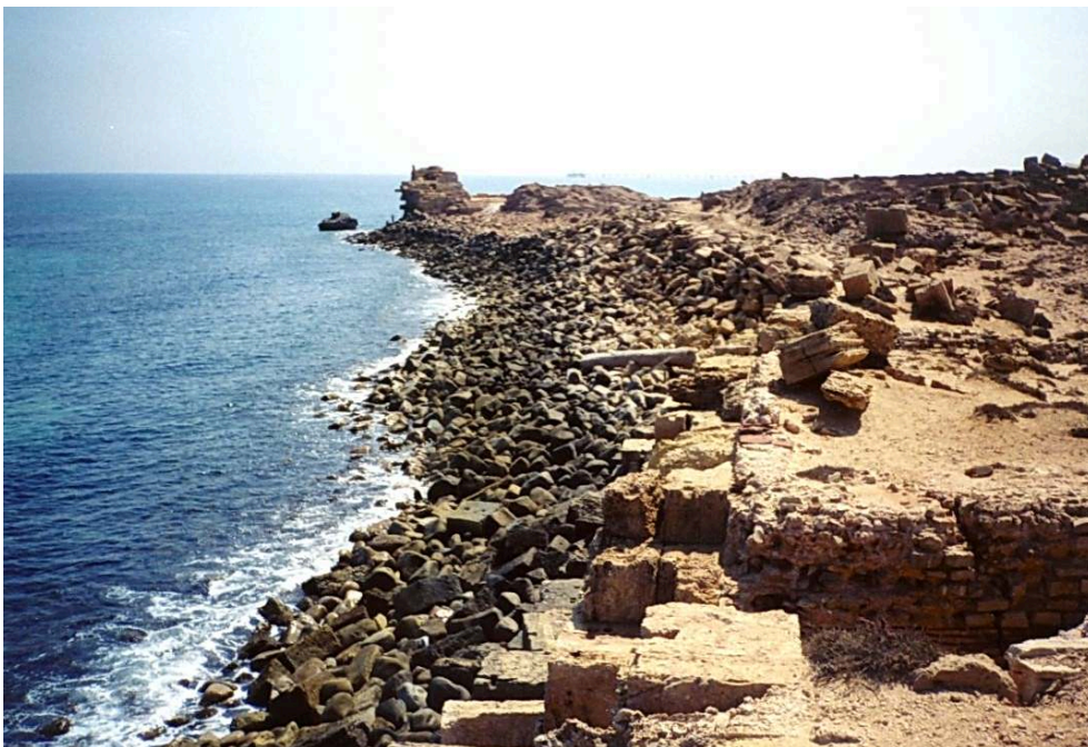
Fig. 32. Berm breakwater on the north coast of Leptis Magna
