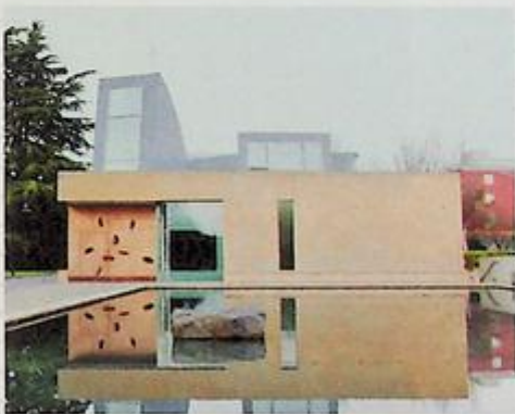
Steven Holl: The Chapel of St. Ignatius, Seattle, Washington, 1997 views of exterior and interior
