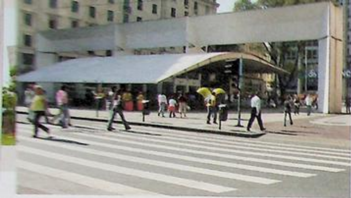
Mendes da Rocha: Underground passage entry on the Patriarch Plaza, São Paulo, Brazil, 1992
