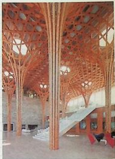
Top: Shigeru Ban: Paper Bridge, Gardon River, France, 2007 Above: Shigeru Ban: Haesley Nine Bridges Golf Club House, Yeosu, South Korea, 2009
