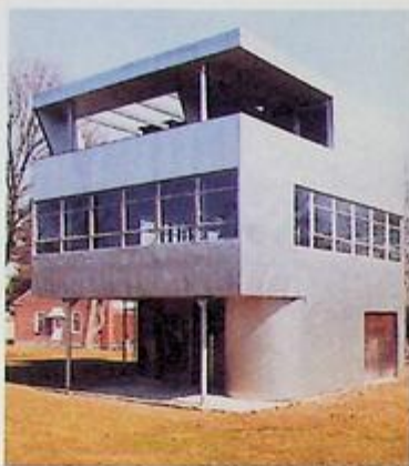
Albert Frey and A. Lawrence Kocher's 1931 Allied and Arts Industries exhibition house Aluminaire was entirely manufactured from existing new materials. Here, form was developed independent of site, with lights that simulated daylight recessed into ceilings and projected
