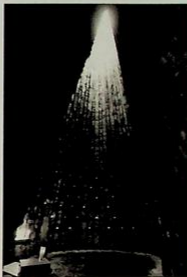
The inner space of the Bruder Klaus Field Chapel by Peter Zumthor in Wachendorf, Germany (2007), was created by burning away the locally forested spruce trees that had been arranged in a
