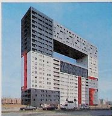
HVRDV's 2001–12 Mirador in Madrid, Spain, takes the typical urban block composed of a series of individual apartment typologies surrounding a collective courtyard space, and conceptually hinges it 90 degrees to create a single vertical neighborhood of connected, yet still distinct, apartment complexes with the former "courtyard" becoming a window that frames the city beyond.
