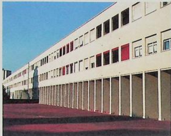
Aldo Rossi: Gallarate II Housing, Milan, Italy 1974 Aldo Rossi's Gallarate II Housing block in Milan takes not only certain formal cues from Giorgio de Chirico's trancelike metaphysical painting, Mystery and Melancholy of a Street , with a giant loggia surmounted by a cadence of square windows, but there is also a similar sensibility of urbanism, of buildings as monumental backdrops that impressively modulate individual activity while suggesting the mysteries that might be hidden in their shadowy depths.
