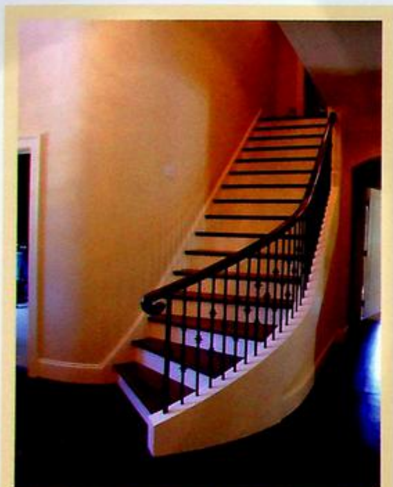
Built of "standard" stair parts, this railing separates itself from the ordinary—but at a reasonable cost.
