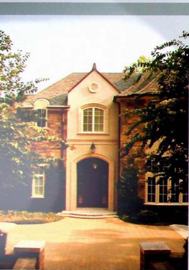
Drawing on classical proportions, this cast limestone entry façade gave this house verticality and an “Old World” dignity not often found in newly built houses.
