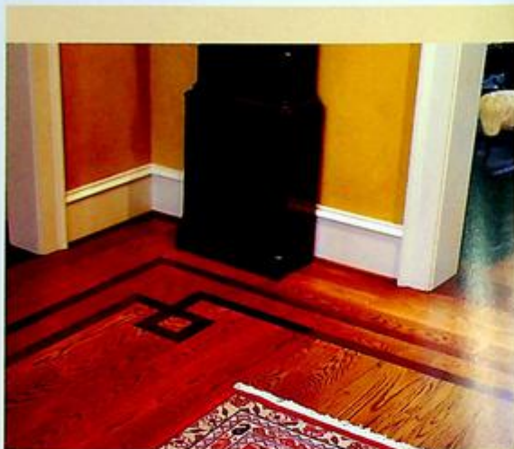
Sapele, a wood species reminiscent of mahogany, is inlaid in a white oak floor. When placing inlays, plan ahead so that they do not end up covered over by furniture or rugs. Open rooms, such as foyers and hallways, are good places for inlays.
