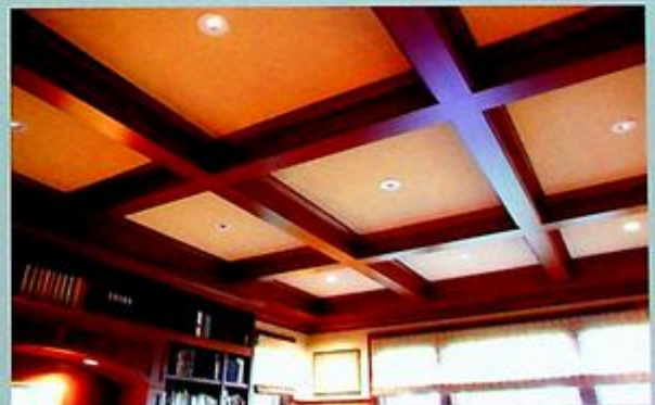
Wood cross-beams create coffers in a library ceiling. Although expensive, beamed ceilings are elegant and wonderful.
