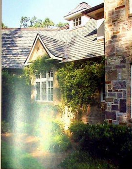
The cupola atop the roof ridge throws natural light deep within the kitchen below. It also adds an interesting feature to the roofline.
