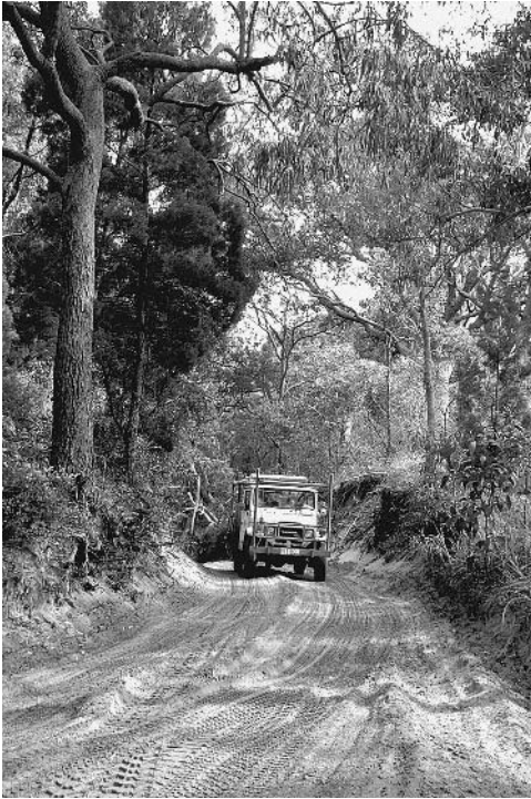
Fig. 7.2. Monitoring involves a programme of impact measurement. A lack of impact standards results in a lack of monitoring. Over time the tourism vehicles eroded away this sand dune in Fraser Island National Park. A lack of erosion impact standards and the resultant lack of impact monitoring allowed much erosion to take place before corrective action was ultimately taken. Road erosion in Fraser Island National Park, Australia. (Photographed by Paul F.J. Eagles.)
