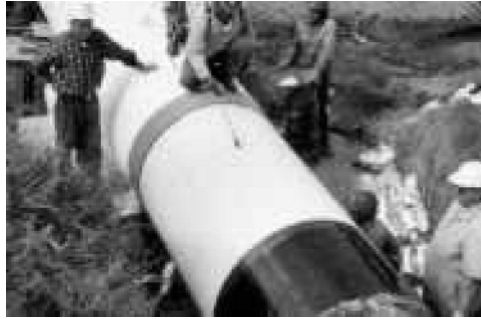
Figure 8. Implementation of strongback sleeve on field.
