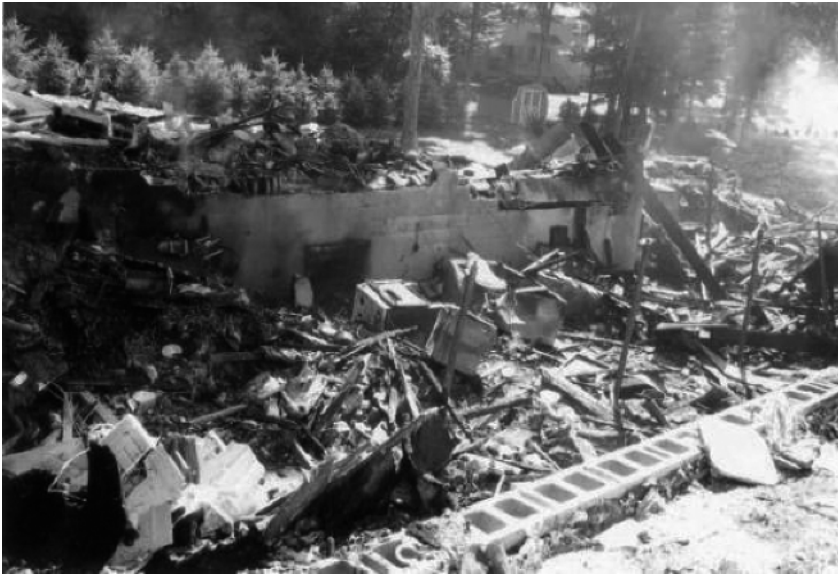
Figure 2. Explosion of gas pipeline in Dubois, Pennsylvania, USA.
