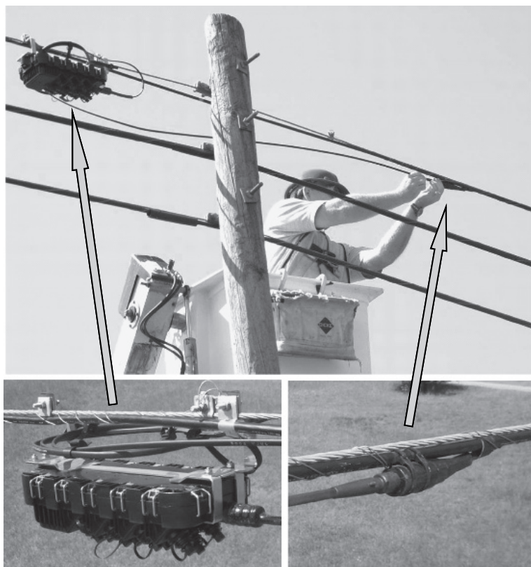
Figure 10.20 Factory installed aerial cable branch point and fiber drop terminal closure (photos) (this figure may be seen in color on the included CD ROM).
