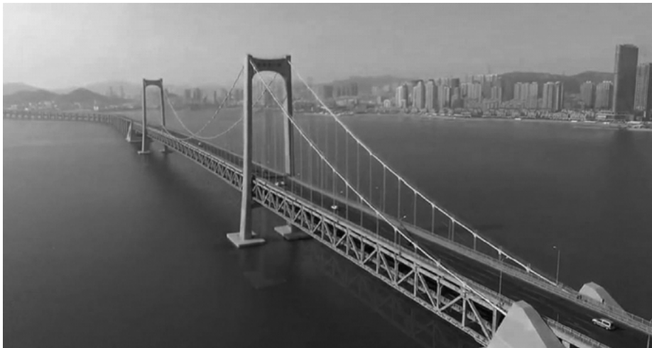
Figure 3.34: Xinghai Bay Cross-Sea Bridge in Dalian (Dalian, China).
