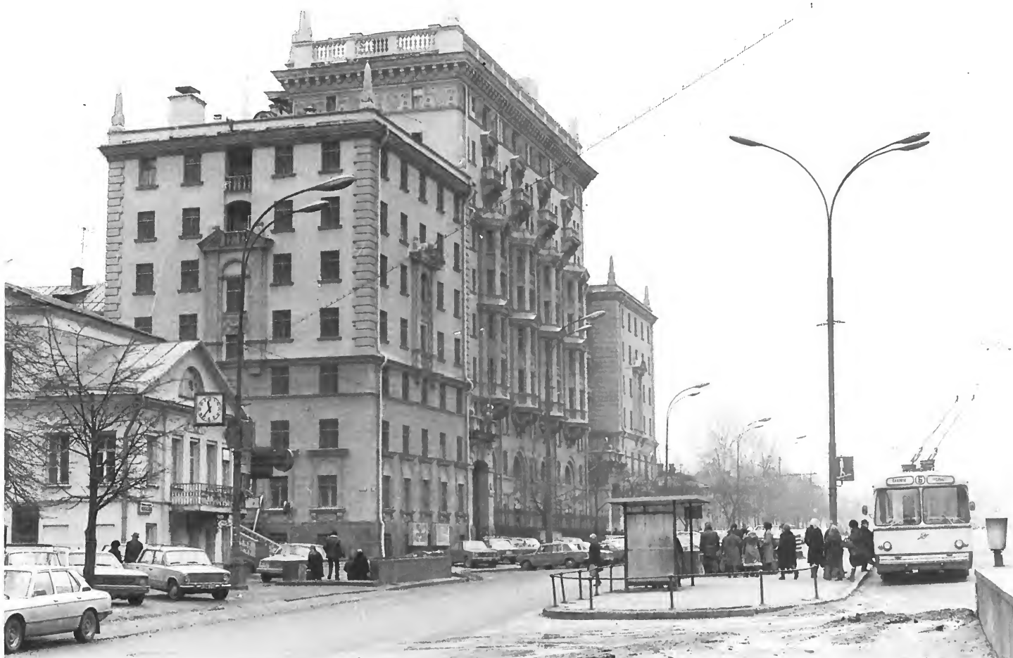
ABOVE: The US embassy building in Moscow. Among the problems encountered by staff there was at one time the bombardment of the building with ultra frequency radiation as part of a Soviet bugging operation, leading to a serious health risk.
