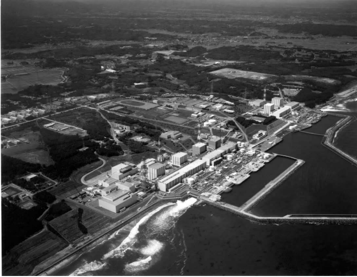
Figure 2.1 The Fukushima nuclear power plant in Japan in 2007. A majority of the world's nuclear power plants are located in the immediate vicinity of the sea. This is because they are in need of massive water supplies. This also makes them highly vulnerable to flooding, as demonstrated most tragically by the disaster at Fukushima in March 2011. Photo: Tokyo Electric Power Co. (TEPCO) / IAEA.
