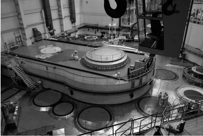
Figure 3.3 IAEA inspectors at work in the Czech Republic, November 2012. The inspectors seal the spent fuel pond, which is situated next to the reactor at Dukovany Nuclear Power Plant. Photo: Petr Pavlicek/IAEA.
