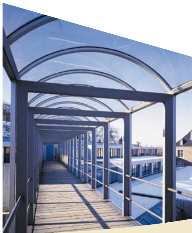
Cintro profiles for barrel vault rooflights
