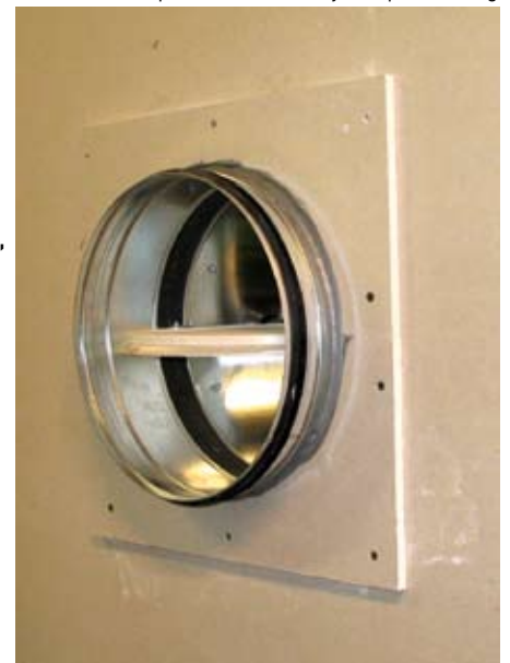
CW60 fire damper mounted in drywall partitioning
