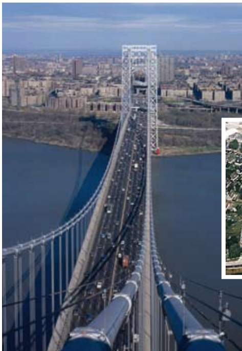
New York George Washington Bridge
