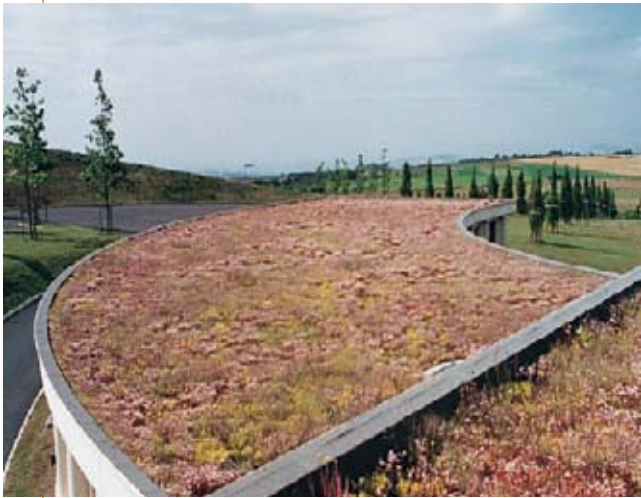
Prevegetated green roof build-up by Soprema
