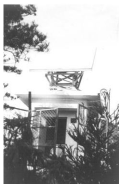
Fig.29: Mt. Shinobu wireless relay station Credit: © NEC
