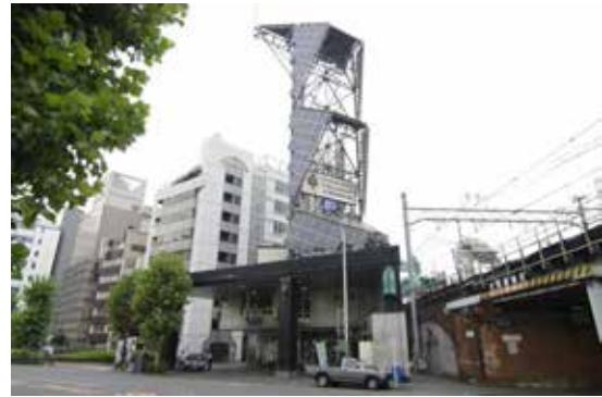
Fig.75: Gas station with solar tower in Tokyo Credit: © Robert Baum
