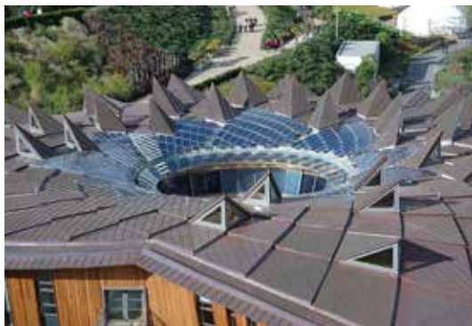
Fig.57: The Core at the Eden Project Credit: © www.solarcentury.co.uk
