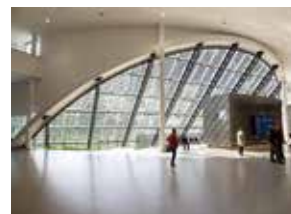
Fig.10: BST - OLV Hospital, 2009 - cs78 Credit: © Sapa Building System
