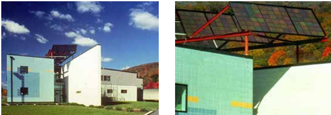
Fig.39 (a) and (b): Chronar PV Port Jervis Factory Credit: © Kiss + Cathcart, Architects
