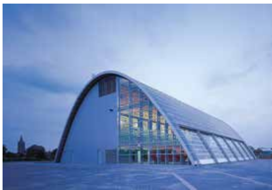
Fig.55: Fire Station Houten Credit: © Christian Richters
