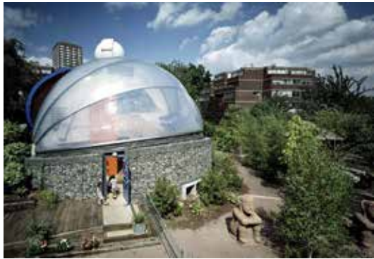
Fig.63: Classroom of the Future Credit: © Studio E Architects
