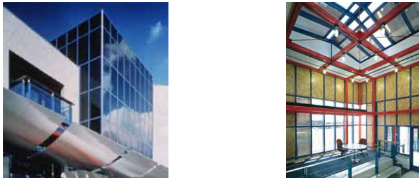
Fig.42 (a) and (b): APS Fairfield PV facility, PV 'cube' and PV skylight Credit: © Kiss + Cathcart, Architects
