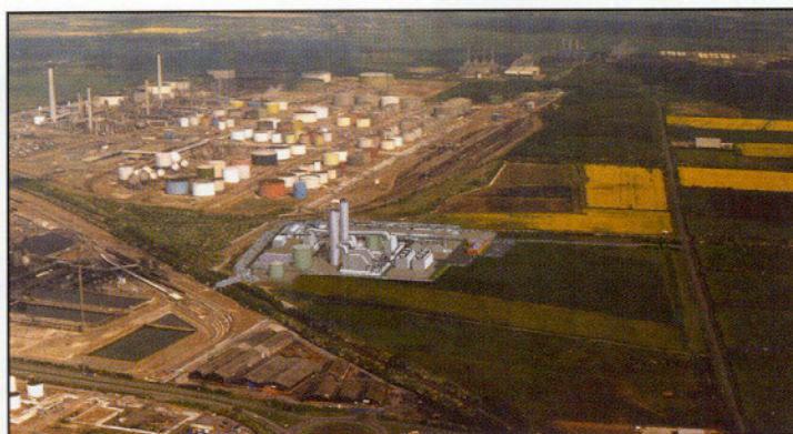
Conoco Global Power Developments UK: State of the Art CHP Plant
